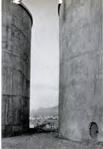
4 Seven circular concrete tanks store hot water on a hill overlooking the capital. Almost boiling at the springs, the water loses only a few degrees on its 10-mile journey.
